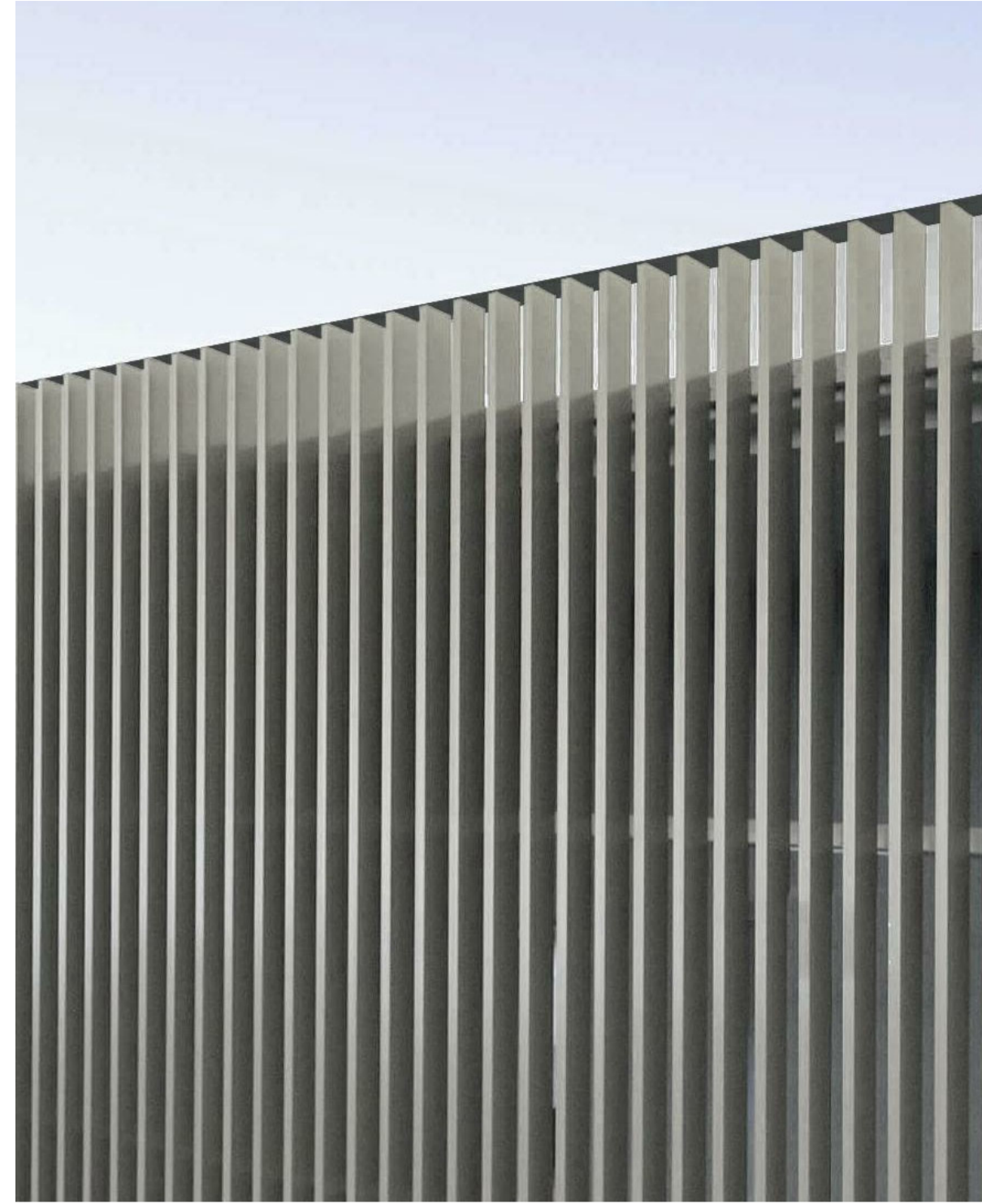
VERTICAL ALUMINIUM BLADES IN MATT POWERCOAT, LIGHT WARM GREY
