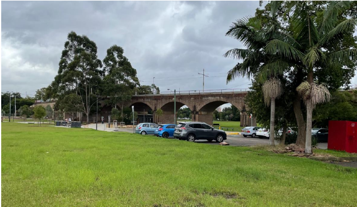
Figure 4: The Railway Viaduct adjoining Chapman Road to the north. View is from the Crescent parklands looking north-east to the viaduct.
