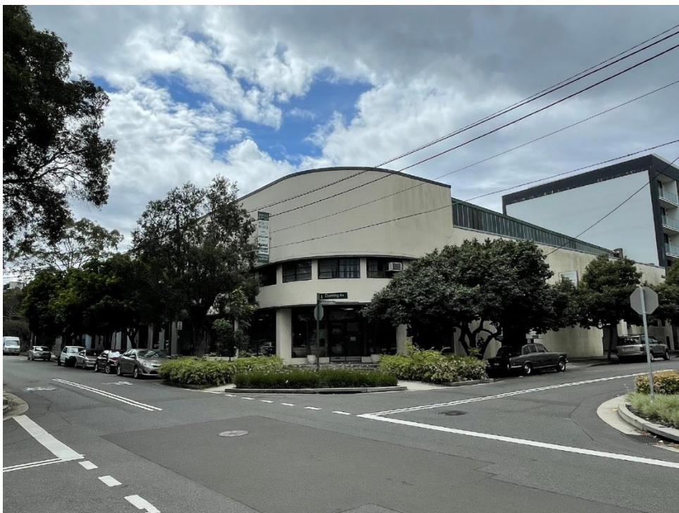
Figure 2: Site viewed from the corner of Dunning Avenue and Cressy Street, looking northeast
