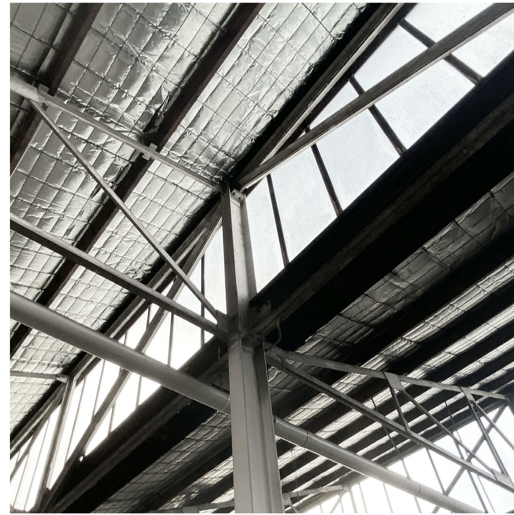
EXISTING INTERNAL HERITAGE TRUSSES AND COLUMNS, REPAINTED WARM MID GREY
