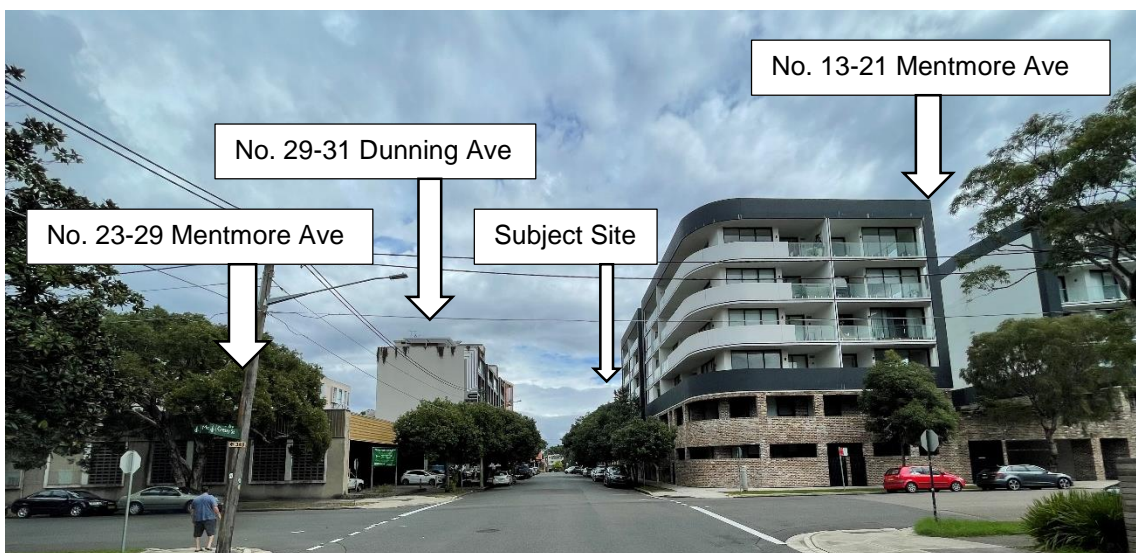
Figure 9: Number 13-21 Mentmore Avenue and 23-29 Mentmore Ave, residential developments to the immediate east of the subject site
